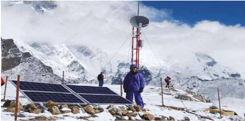
Figure 2: NWNP tower is installed in a Nepalese peak of the Himalayas 258 .
